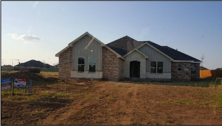
Figure 7: South Abilene Area New Home Construction
